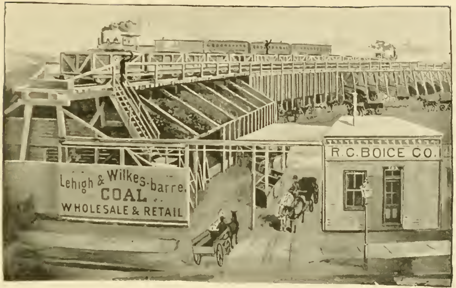
YARD AND ASH PIT OF THE R. C. BOICE COMPANY, MARKET STREET AND CENTRAL RAILROAD.
